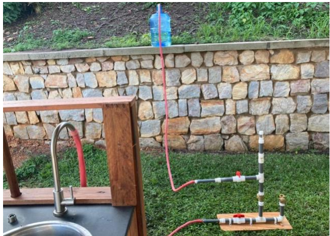
Fig.12 – Completed ram pump filling dispenser tank
